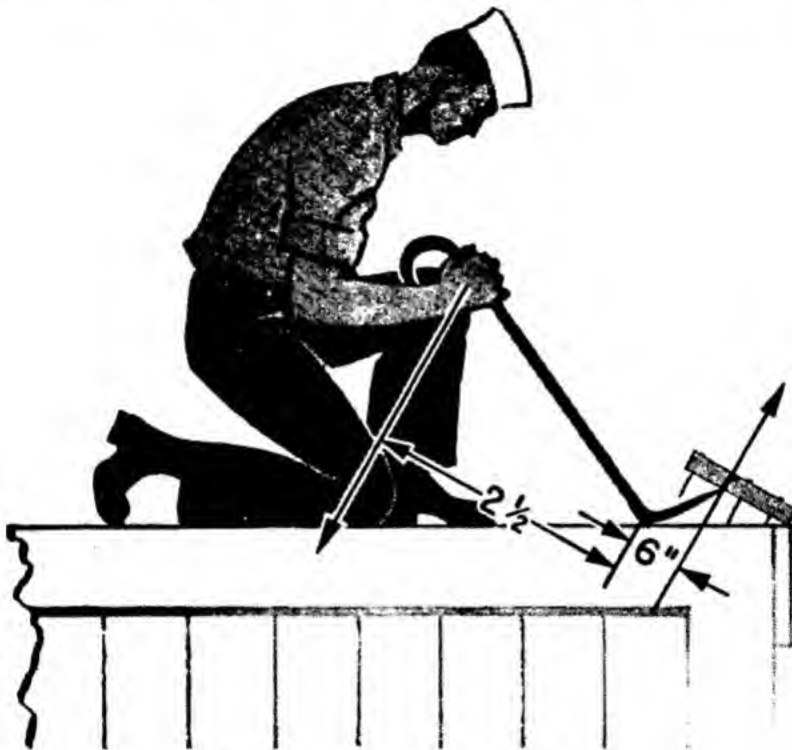
Figure 11.—Using a wrecking bar.
